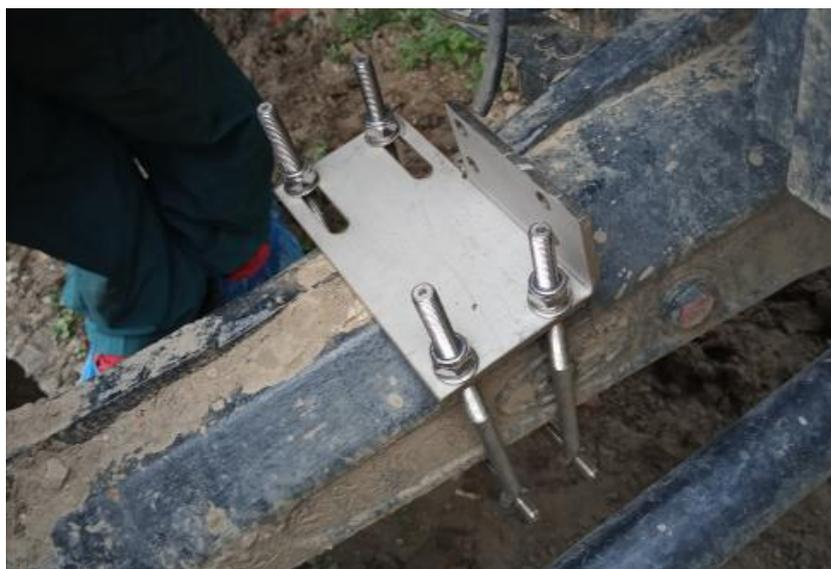
Figure 2.8 Install the parts to fixate angle sensor
