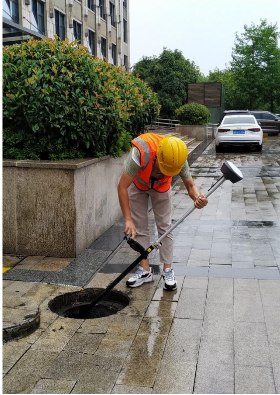
Figure 5.5 Tilt survey for a manhole
