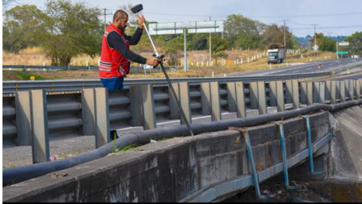
Figure 5.2 Tilt survey– on the bridge
