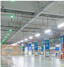
Indoor structures, underground parking area
